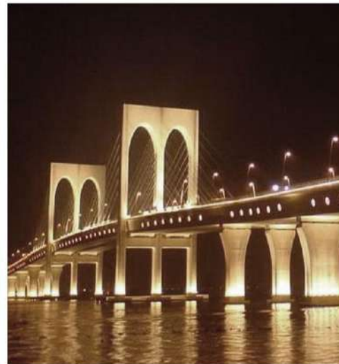
Bridge lighting-Warm white
